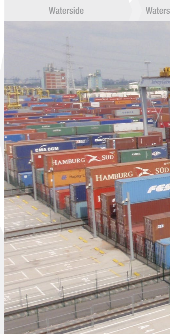
Automated Stacking Cranes – Antwerp Gateway, Belgium
