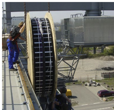
Energy guiding chain assembly on an intermodal crane
